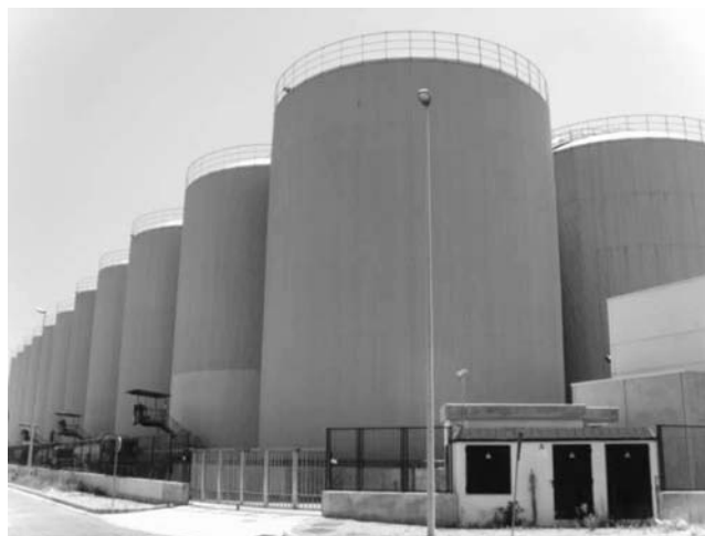
FIGURE 52.12. Storage tanks in Barcelona, Spain, constructed of S32101.
