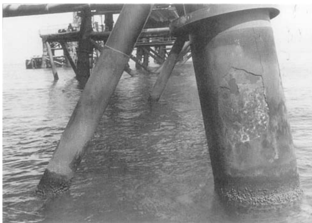
FIGURE 68.2. Splash zone coating damage and corrosion on offshore platform. (Photo furnished by Lone Star Corrosion Services, Lancaster, TX.)
