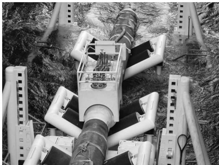
FIGURE 87.18. Ring pair corrosion monitoring system being deployed at sea during the installation of a submerged pipeline. (Courtesy of Cormon Ltd.)
