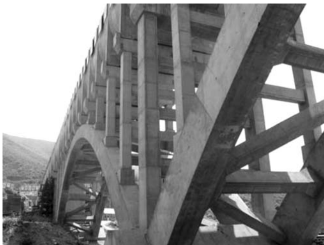
FIGURE 32.7. Photograph of an open aqueduct structure under construction for drinking water transport from mainland China to Hong Kong.
