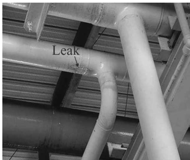
FIGURE 50.1. SCC observed in terminal piping system containing FGE.
