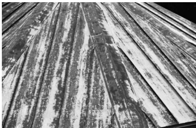
FIGURE 1.3. Terne-coated roof showing severe reddish-yellowish discoloration instead of the expected gray patina.
