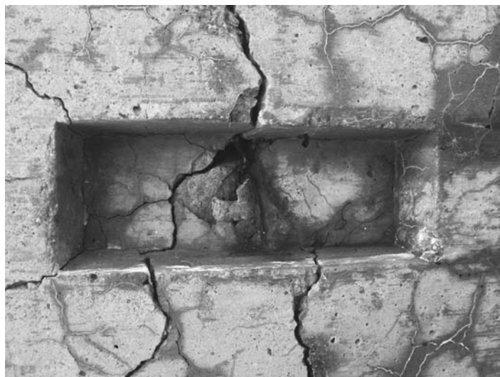
FIGURE 23.6. Cracking of concrete cover in marine environment. (Courtesy of Kingston Technical Software.)
