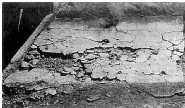
FIGURE 31.5. Disintegration of concrete caused by sulfate attack [9].
