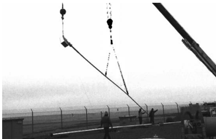
FIGURE 87.15. Installation of first full-scale probe into a double-shell tank (DST) at the Hanford site. (Courtesy of HiLine Engineering & Fabrication.)
