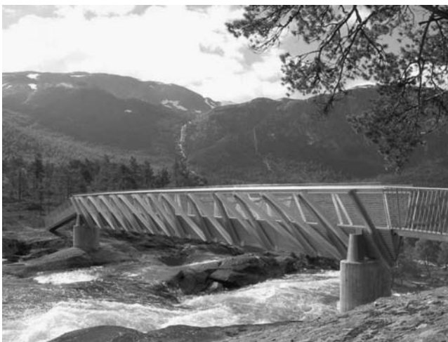
FIGURE 52.13. Walking bridge in Norwegian mountains constructed of S32101.
