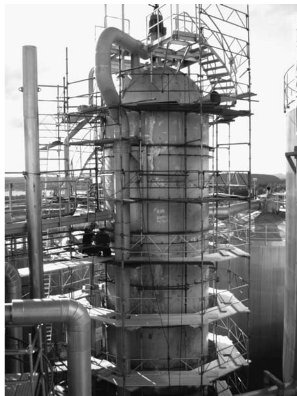
FIGURE 52.11. Peroxide reactor in S32101 for pulp and paper mill.
