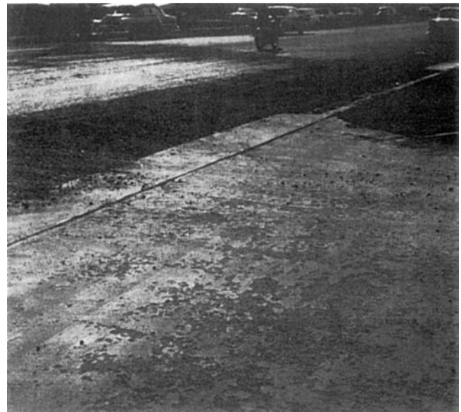
FIGURE 31.2. Surface scaling of concrete caused by deicing chemicals [6].
