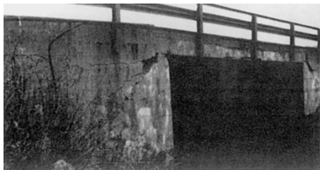
FIGURE 31.3. Cracking in a concrete bridge caused by alkali-silica reaction [8].
